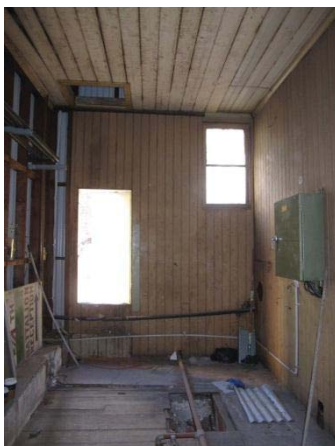
FORMER LIFT MOTOR ROOM/ PLANT ROOM BETWEEN THE GABLES.
