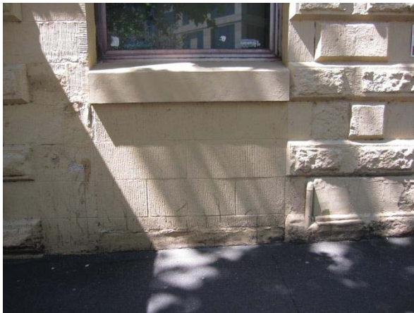
DETAIL OF THE INFILLED CENTRAL ENTRY (12) AND SANDSTONE QUOINING.
