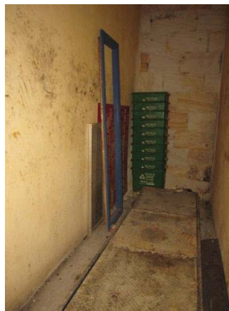
REAR SERVICE AREA – VIEW TO NORTHERN STORE WALL
