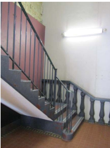
GROUND FLOOR STAIR HALL WITH CONCRETE STAIR AND METAL BALUSTRADE
