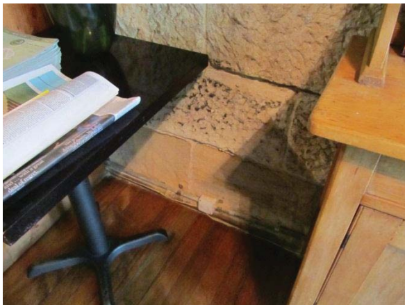
DETAIL OF THE SOUTHERN STORE WALL AND TIMBER FLOORING
