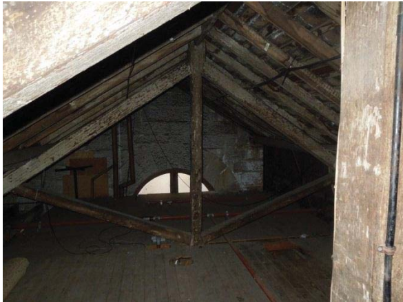
VIEW OF THE KING POST TRUSS AND EASTERN GABLE
