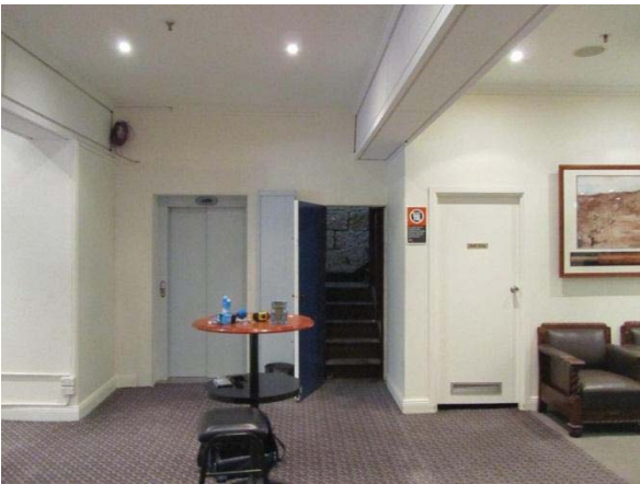
VIEW NORTH SHOWING THE ROOF ACCESS STAIR, LIFT AND ACCESS TO WC
