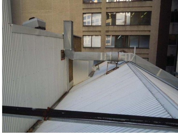
VIEW EAST OVER THE SOUTHERN STORE GABLE AND ROOF ADDITION
