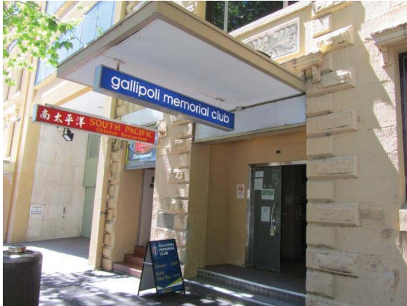
GROUND FLOOR NORTHERN STORE (12 LOFTUS STREET) SHOWING THE NEW OPENINGS AND AWNING.
