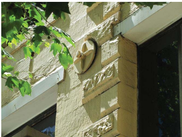
STRUCTURAL REINFORCEMENT OF THE WESTERN FAÇADE
