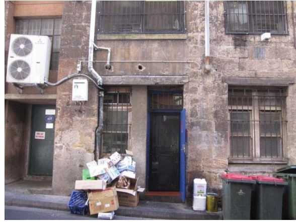
GROUND FLOOR OF THE SOUTHERN STORE (14) SHOWING LATER OPENINGS
