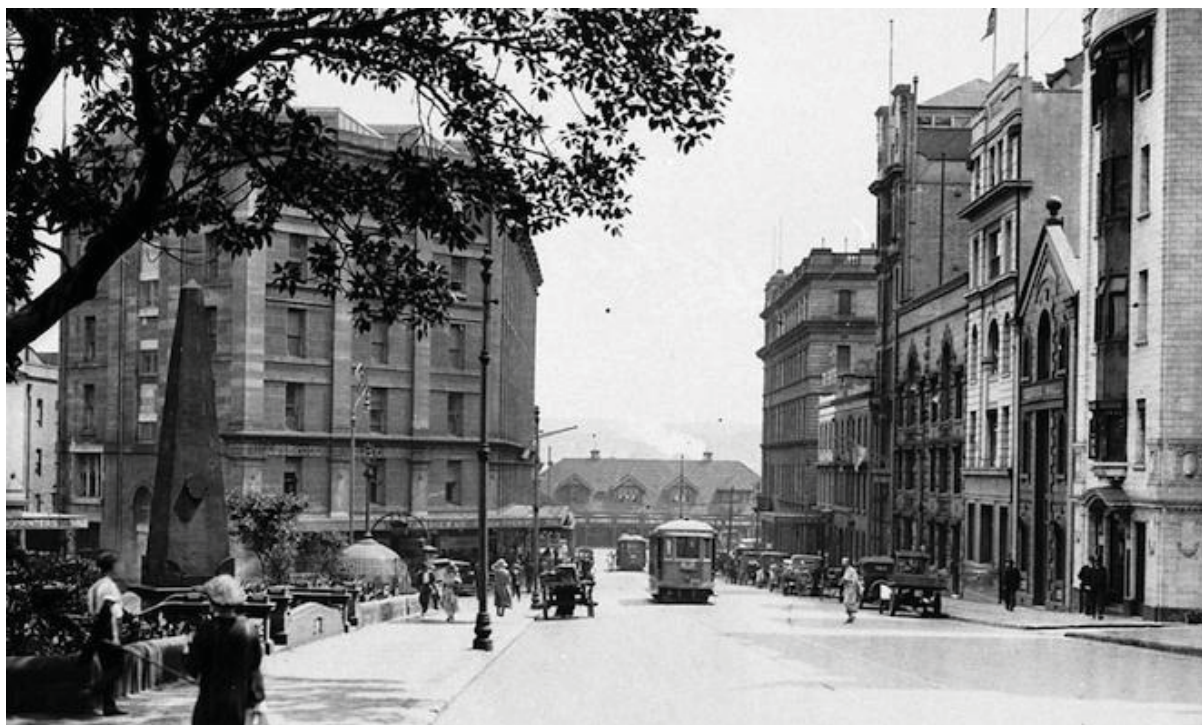
FIGURE 38 – MACQUARIE CHAMBERS IN THE STREETScape
