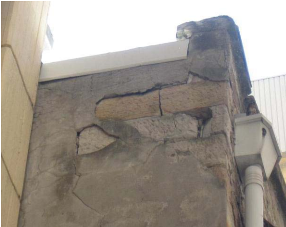
FIGURE 11 – THE SOUTHERN RETURN/ LOFTUS LANE
