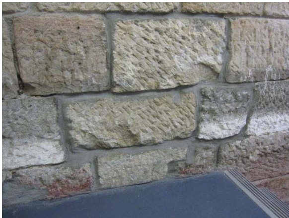
DETAIL OF CEMENT POINTING TO LEVEL 2 STONEWORK
