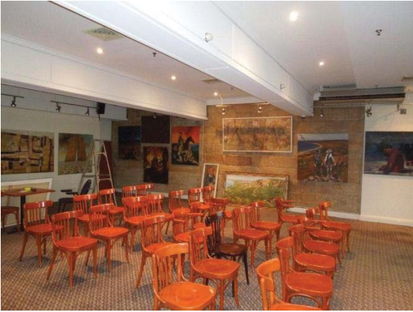
THE BOARDROOM VIEW SOUTH TO SANDSTONE WALL. THERE IS POTENTIAL FOR ORIGINAL CEILING BEAMS TO BE RETAINED WITHIN THE FALSE BEAM STRUCTURES
