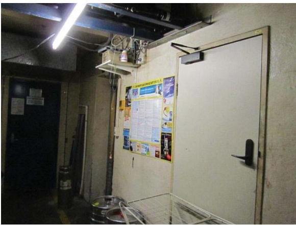
REAR SERVICE AREA - COOL ROOM AND GREASE TRAP
