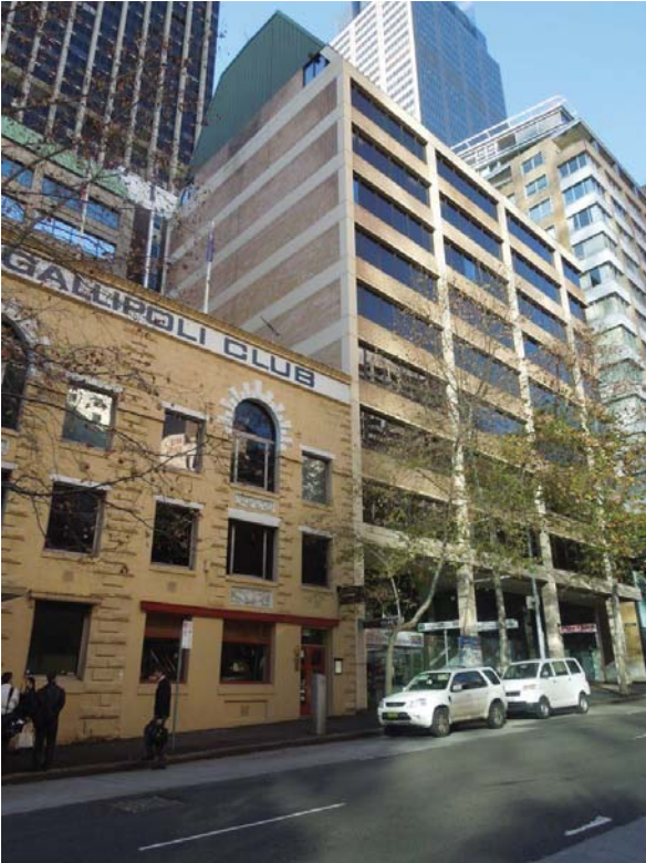
THE SUBJECT SITE (LEFT) AND ADJOINING 10-11 STOREY COMMERCIAL BUILDING AT 16-20 LOFTUS STREET
