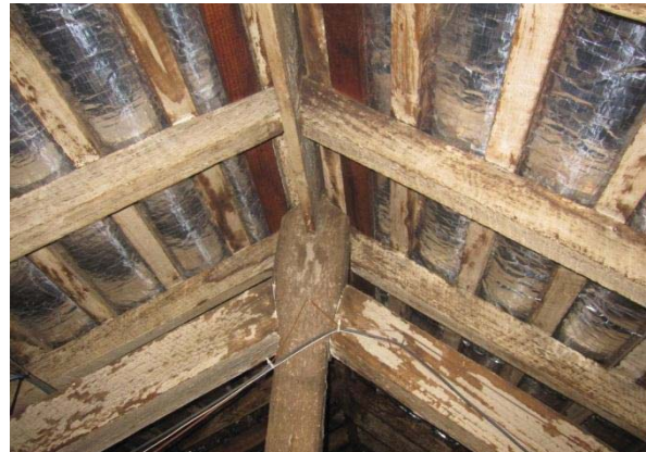
DETAIL OF CEILING BATTENS (THE PLACEMENT OF WHICH INDICATES A FORMER SLATE ROOF)
