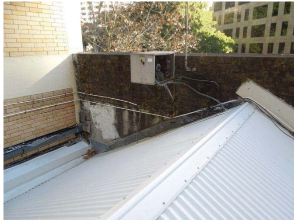
THE INTERNAL FACE OF THE LOFTUS STREET PARAPET
