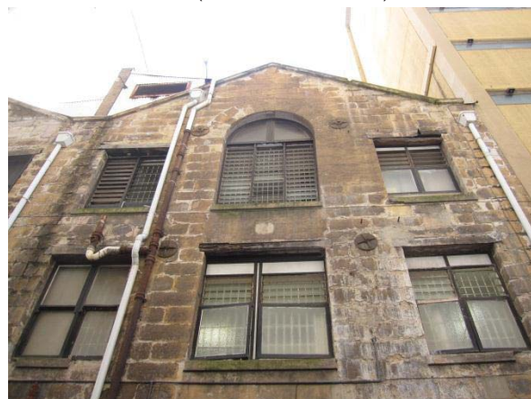
DETAIL OF THE NORTHERN STORE FAÇADE SHOWING THE INFILLED SPANDRELS WITHIN THE CENTRAL BAY. THE FIRST FLOOR SOUTHERN WINDOW (SHOWN AT LEFT) LIKELY REFLECTS THE ORIGINAL FABRIC AND CONFIGURATION
