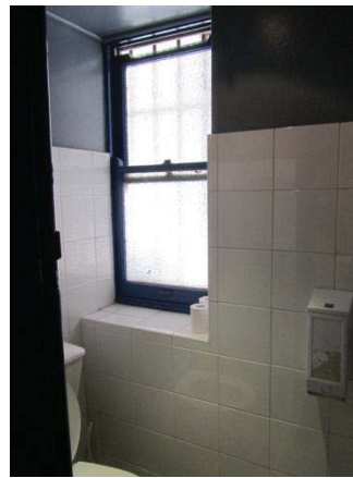
CONTEMPORARY WC FIT OUT
