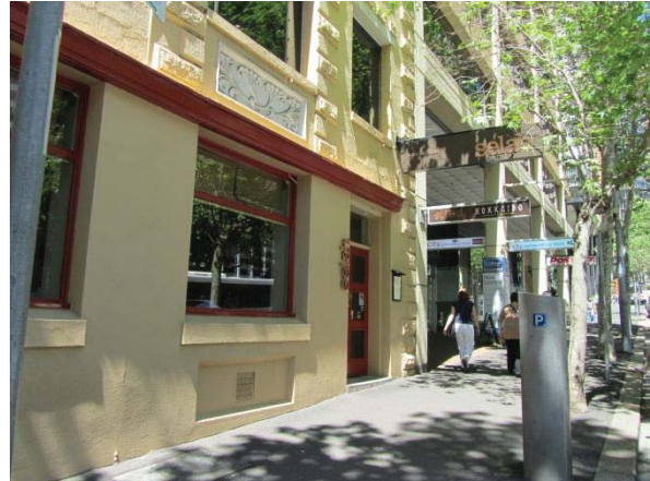
GROUND FLOOR SOUTHERN STORE (14 LOFTUS STREET) SHOWING THE C.1910 ENTRY AND REMNANT TIMBER WINDOW FRAMES. THE ORIGINAL QUOINS AROUND CENTRAL BAY HAVE BEEN REMOVED
